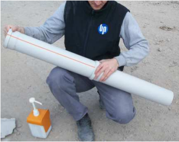
Assembling of pipe
