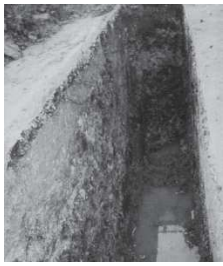
Water should not be left in the trench
