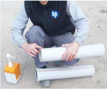
Applying liquid soap on spigot.
