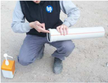
Applying liquid soap on gasket
