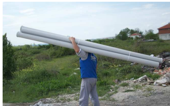
Carrying pipes in bundle at installation site
