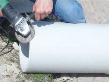
Beveling end of PVC pipe
