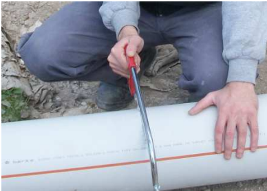
Cutting PVC pipe in the field
