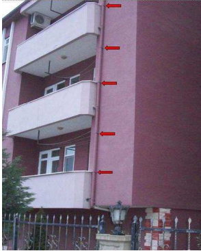
Correct applied clamps.
